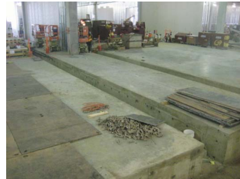
Figure 11 - View of the SOG with Trenches
