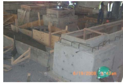
Figure 15 - Cast-in-place UPS pits
