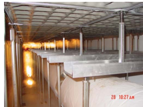
Figure 13 - Bridging over the chilled water pipes
